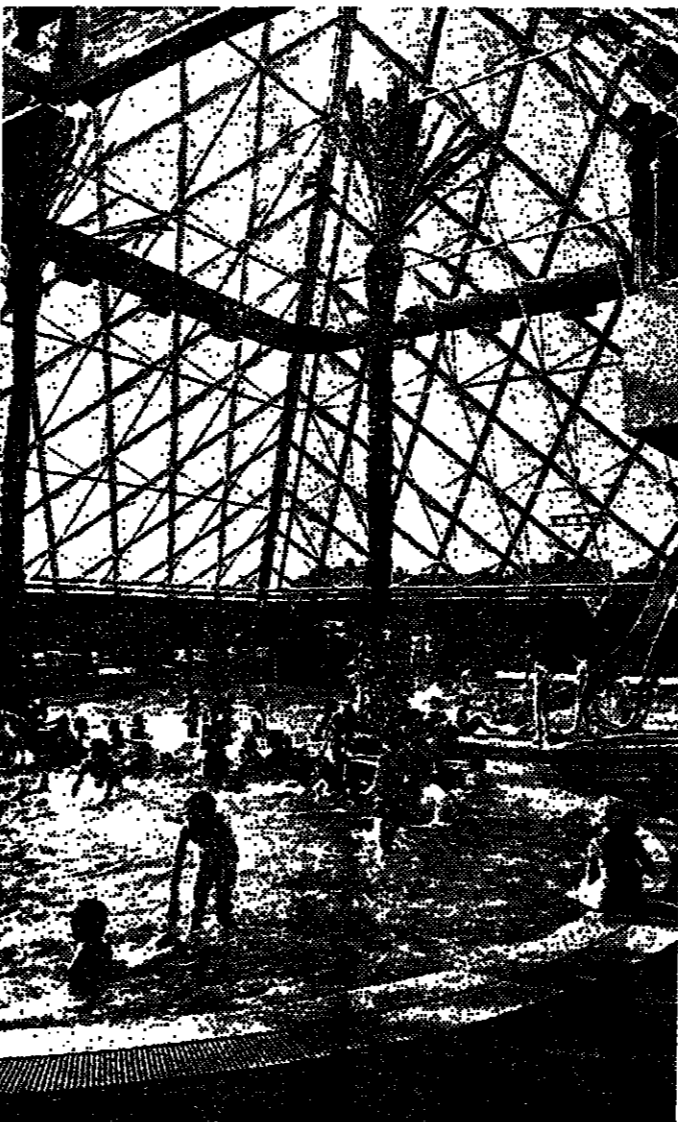
Bothers in the pool at Bleckley Leisure Centre: one of two built as an integral part of the Milton Keynes philosophy that play is as important as work. Each has a theatre and extensive facilities for sport.
